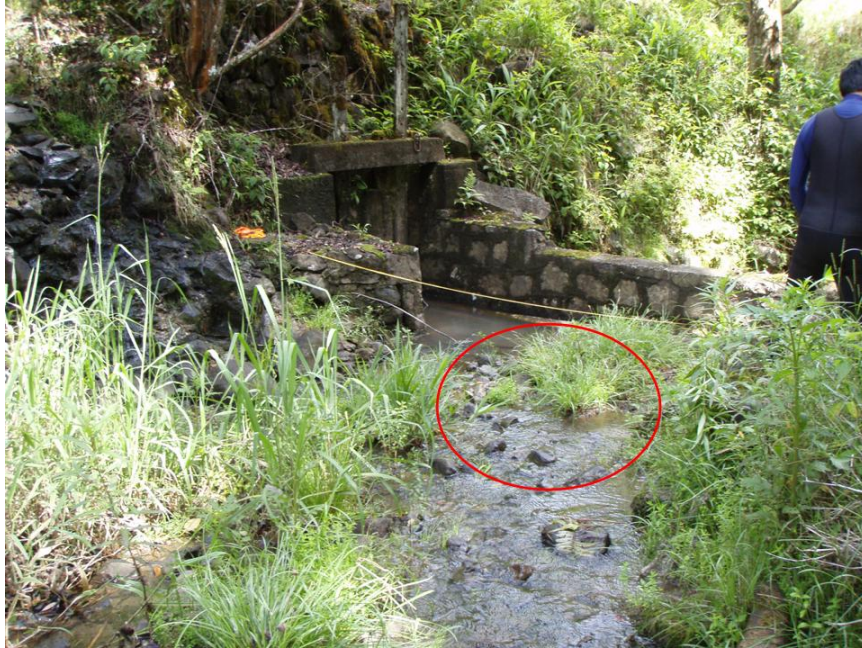
Figure 5-13. Photo is taken facing downstream toward the diversion and survey site 2. (6/30/2009; Tributary name: Nua'ailua (64010001); PBN: In002p-004-063009; Surveyor: Kuamo'o, D.; SBN: dk002d-063009; Lat. (DD): 20.83374, Long. (DD): -156.17751).
